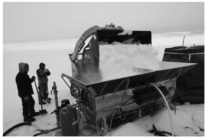
Fig. 6. Caterpillar 297 skid steer loader feeding snow into the melter.
