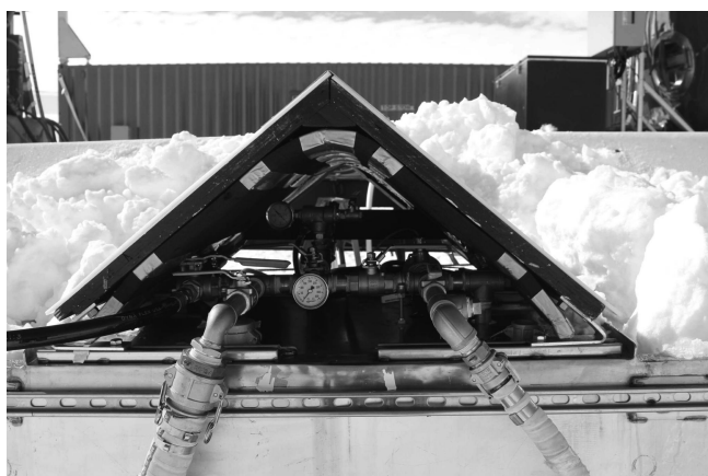
Fig. 5. Operator's view of the tank manifold system shown in the melt tank water-plumbing diagram.
