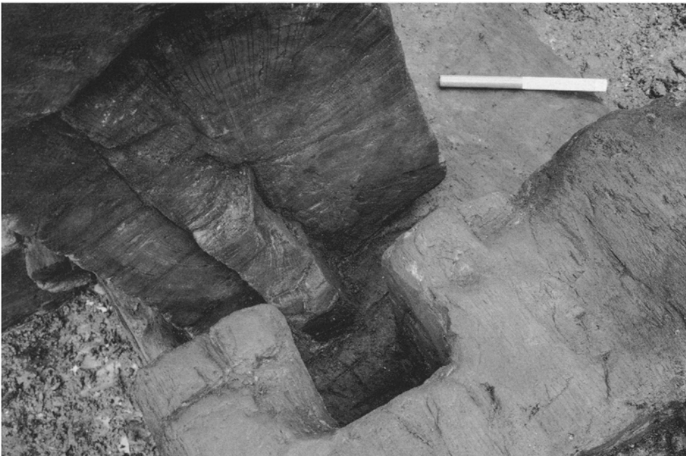
B. Billingsgate: detail of tongue-and-groove scarf joint from the second tier. Scale 2 \times 100 mm. (p. 101).
