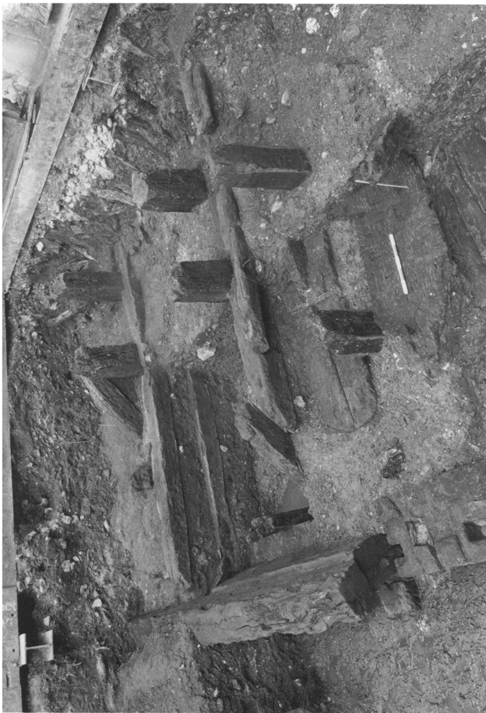
Billingsgate: view of the quay structure with angle braces and tiebacks in place. The angle braces would have prevented the tieback piles from being pulled forward. Scale 5 × 100 mm. (p. 103). (Photo: Museum of London)
