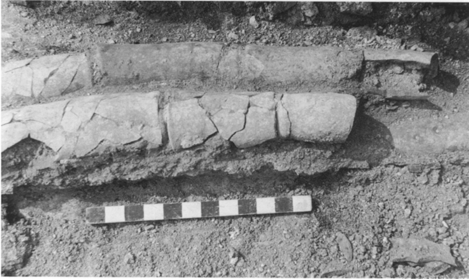
A. Fortress baths at Chester: close-up view of fallen vault-rib of tubuli lingulati . (Scale in inches). (p. 217)
