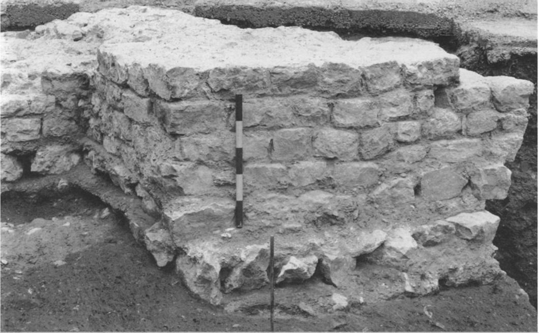
A. London Basilica, second century: Area S, looking E. Buttress on masonry wall representing first phase of construction, dividing Rooms 5 and 6. The 5 \times 100 mm scale rests on off-set foundation which is not separated from superstructure by tile course: cf. PLS. XA and B. (p. 58)
