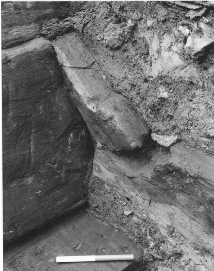
B. Billingsgate: tieback attached to the quayfront using a half-dovetail joint. The joint has failed, allowing the quayfront (left) to subside. Scale 2 \times 100 mm. (p. 102)
