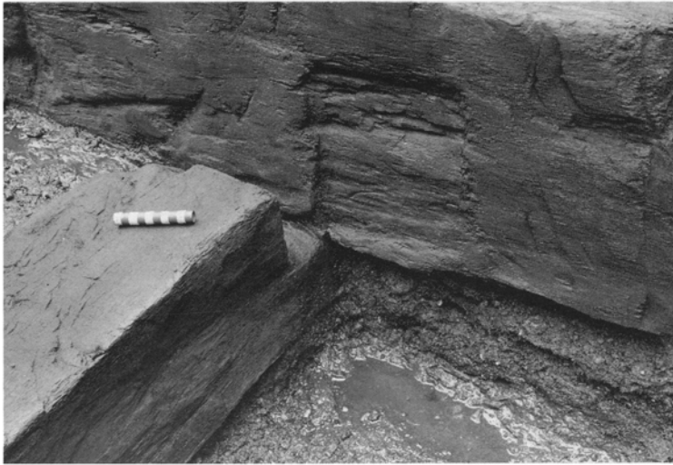
A. Billingsgate: impression left by an angle brace on the rear of a sillbeam, with (left) the cradling timber seen in PL. XVIIA passing beneath the quayfront. Scale 10 \times 10 mm. (p. 102).
