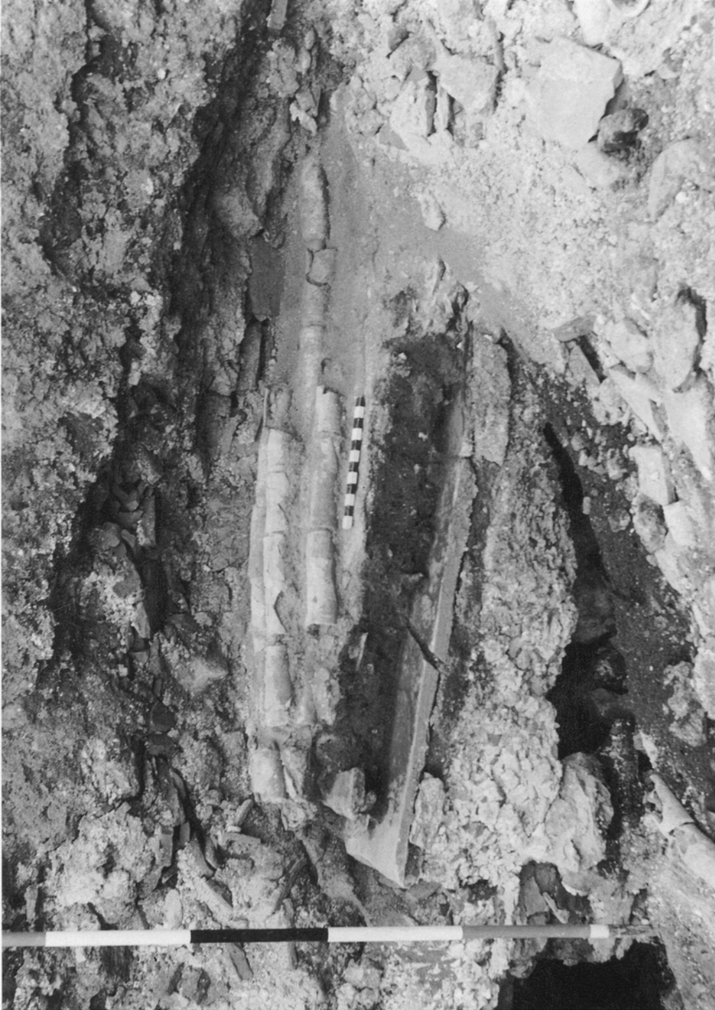
Fortress baths at Chester: fallen section of concrete vaulting seen in 1964 resting on soil accumulation over tepidarium floor. Note the vault-rib formed of lines of interlocking tubuli linguati . (Scale in feet). (p. 217)
