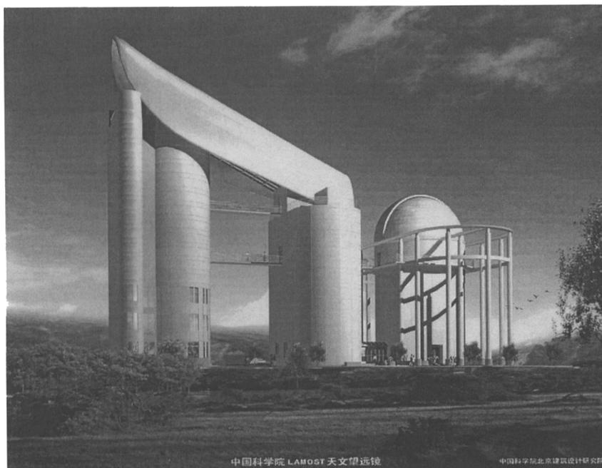
Figure 3. An artist's-eye view of LAMOST. The reflecting Schmidt plate is located in the lower dome on the right-hand side of the plot (south). The spherical primary mirror is on top of the higher tower, which is about 44 m from the ground. The central block is for the focal surface and the spectrograph room. Courtesy LAMOST team
