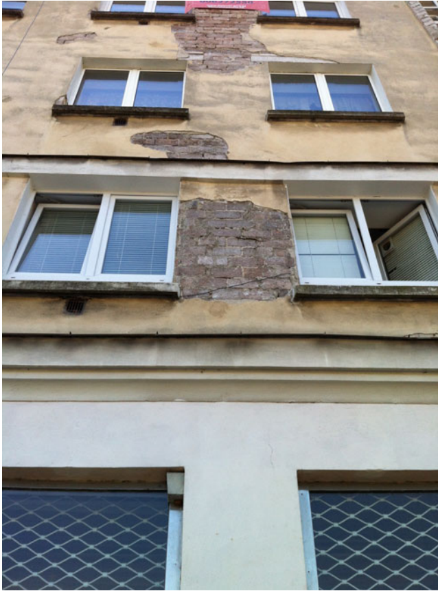
FIGURE 3 Few up-close, color photos of Lachert's red-brick façade exist. However, the social-realist plaster of the 1950s is now peeling off. Photo by Michael Meng 2014.
