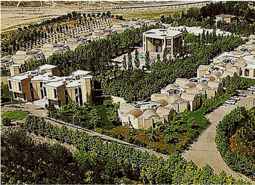
Figure 1. Iran Center for Management Studies, Tehran. Photo courtesy of Nader Ardalan.
