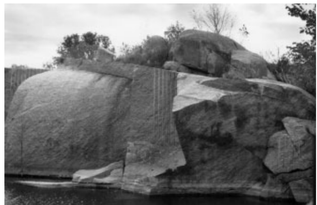
Fig. 5. Site 1b. Recent sheeting of granite resulting from quarrying that has exposed a fresh, parabolic rock surface.
