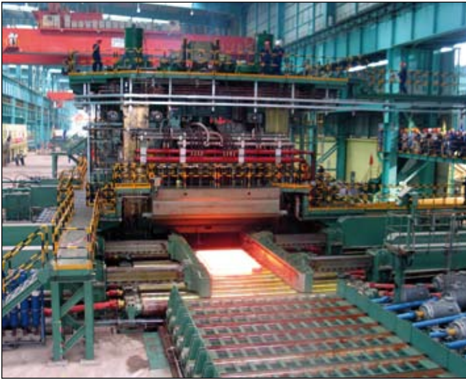
Siemens engineered and supplied key process technology for the new Xiangtan Iron & Steel two-stand plate mill. Photo courtesy of Siemens VAI
