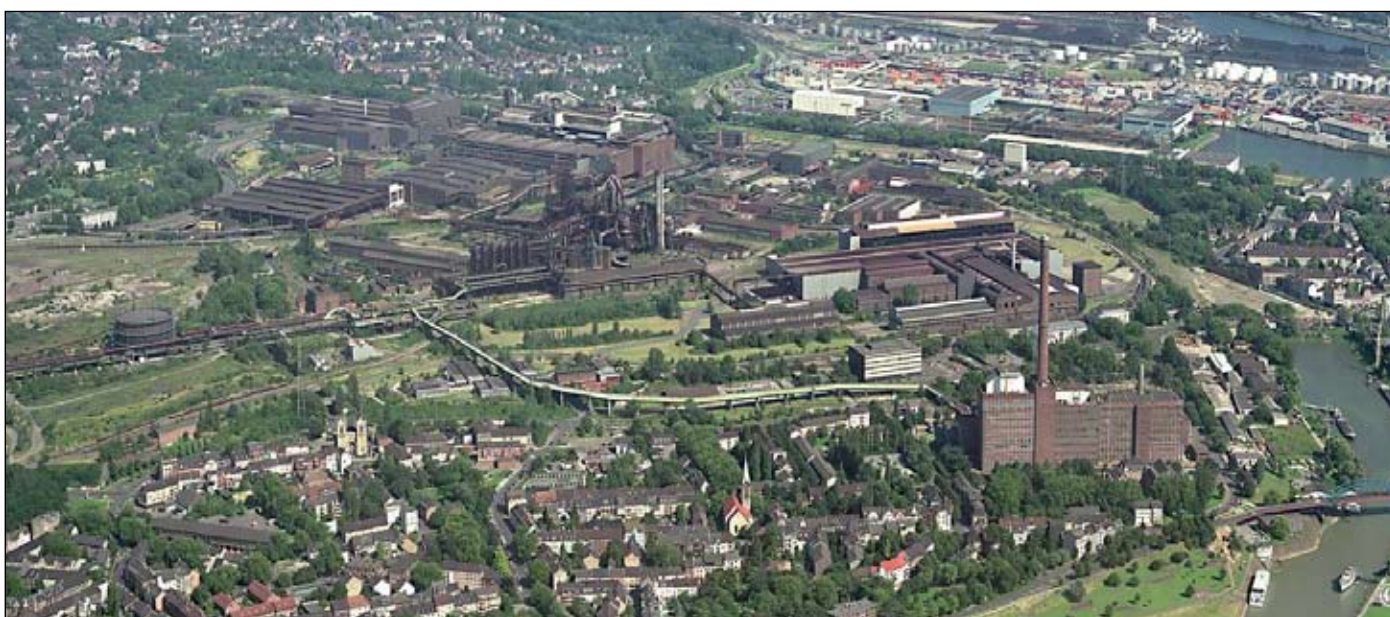
The new wire rod mill is due to start production in spring 2012. Photo courtesy of SMS Meer
