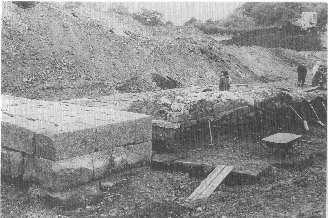
B. Piercebridge: the bridge under excavation showing the later causeway and its surface of limestone slabs. (p. 124)
