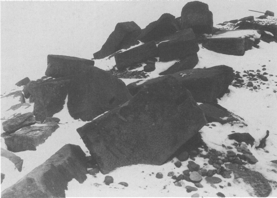
A. Piercebridge: tumbled masonry at Pier 3. In the foreground is a stone with a clamp-socket, beyond is the cutwater from the upstream face with a lewis-hole in its upper surface. (p. 122)
