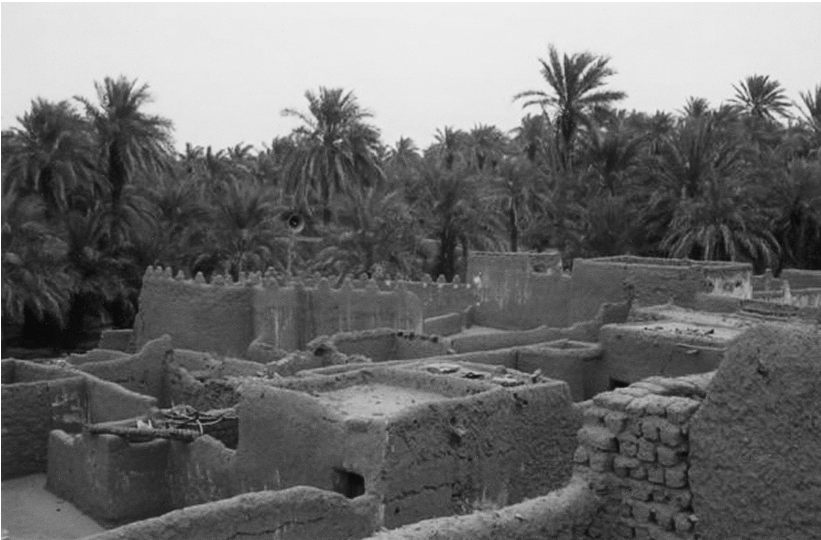
Figure 1.2 View over rooftops of a ksar in the Gourara, near Timimoun (T. Sahrawi).
