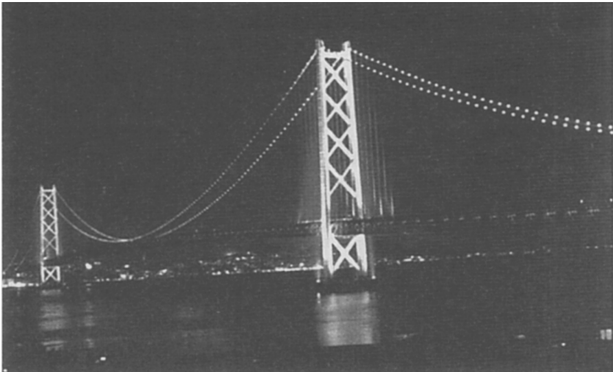
Figure 5. The new Akashi Kaikyo Bridge near Kobe, Japan. Floodlights illuminate only the two towers, each 300 meters (984 feet) high, just equal in height to the Eiffel Tower.
