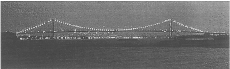
Figure 3. The Bronx-Whitestone Bridge, linking the boroughs of Bronx and Queens in New York, shows the necklace or tracer lights that are in common use throughout the city's many suspension bridges.
