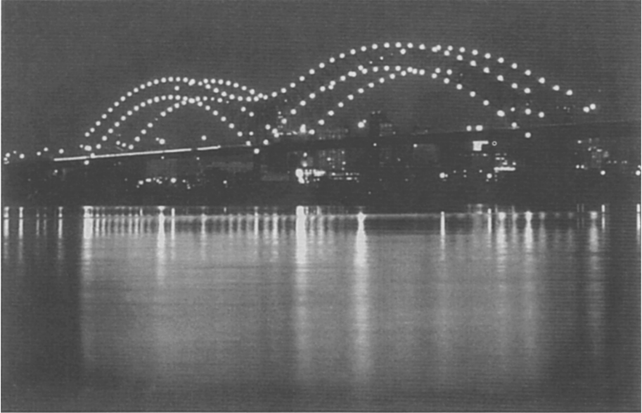
Figure 2. Hernando DeSoto Memorial Bridge at Memphis is a near twin of the Arrigoni Bridge and served as a model for the lighting plan. The 200 tracer lights are HPS 6300 lumens each. There are no floodlights.
