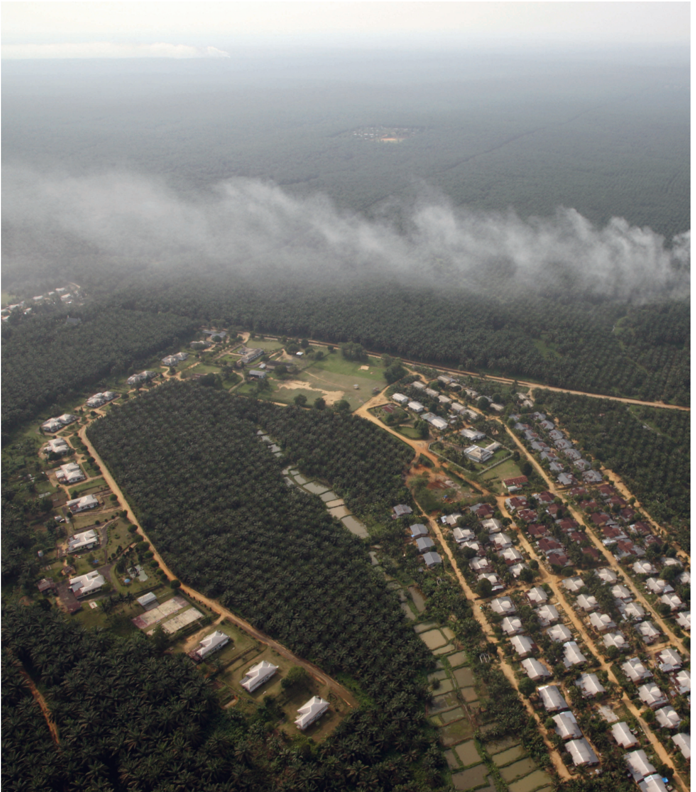
Photo: Palm oil accounts for 40% of the vegetable oil produced worldwide. Palm oil facility, Indonesia. © Greenpeace/John Novis
