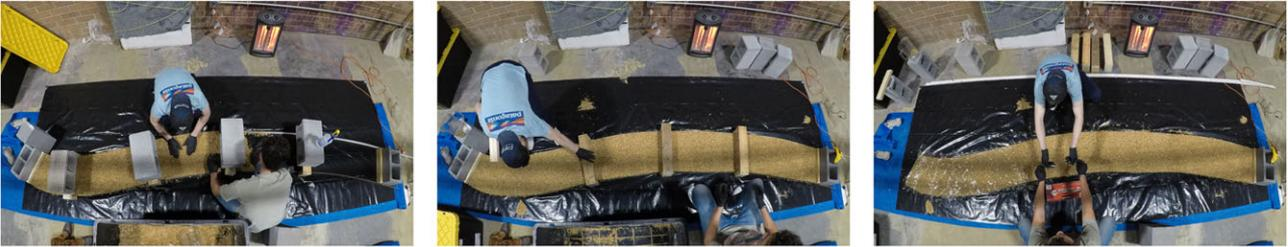
**Figure 6.** In step 2, the formwork is packed with living myco-materials. Photos by Jonathan Dessi-Olive.
