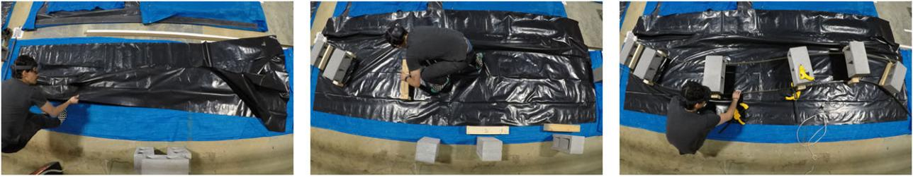
**Figure 5.** In step 1, formwork is laid out on an impermeable membrane. Photos by Jonathan Dessi-Olive.
