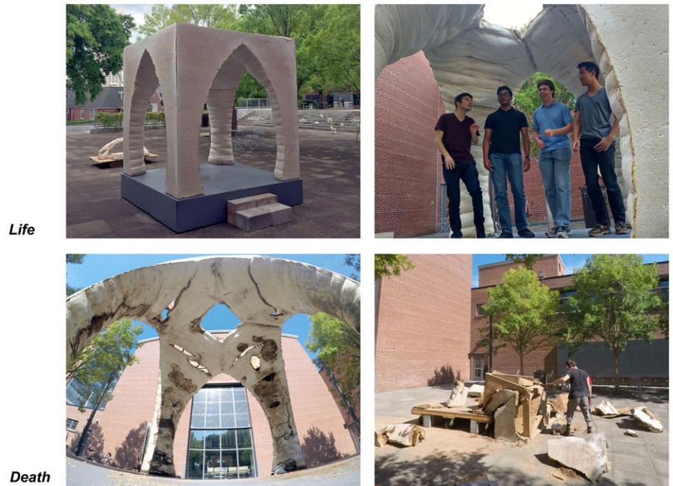
**Figure 1.** Life and death of Monolito Micelio: a monolithic pavilion for a singing performance in May 2018. The structure was cultivated from a single colony of mycelium in a hemp substrate. After the performance, the structure was left to decay and eventually broken down, disposed and “fed” to compost. Photos by Jonathan Dessi-Olive.
