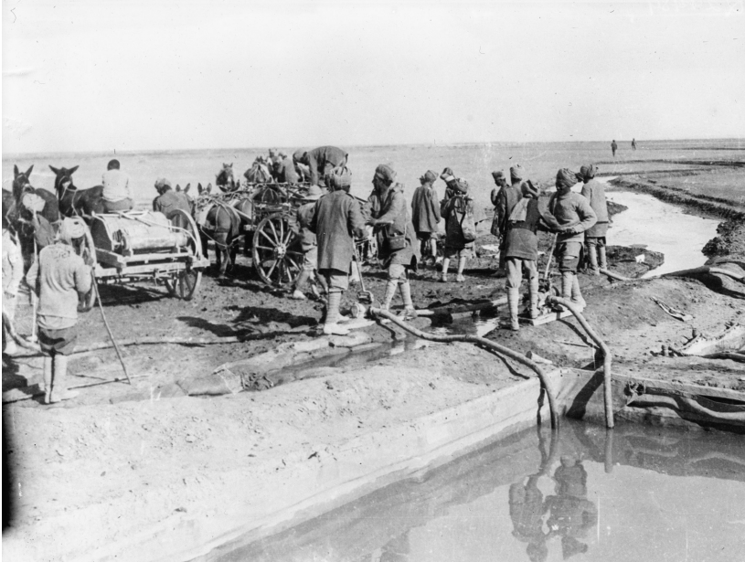
Figure 6.3 Indian army engaged in chlorinating water at an advanced post in Mesopotamia, 1917. © Imperial War Museum (Q 24489).
