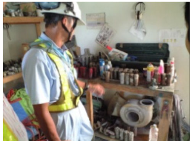
Fig. B2. The spare parts at a tunnel construction site.
