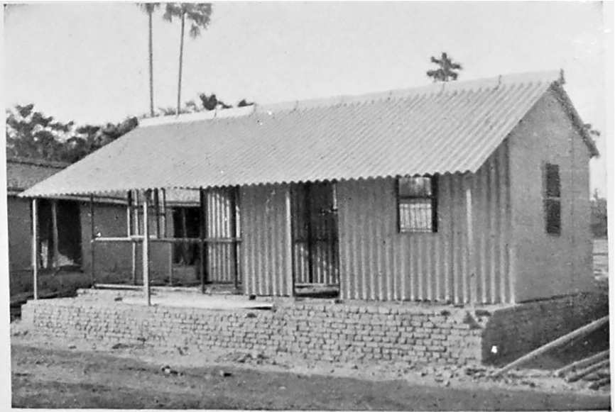
Image 6.7 A demonstration building made of asbestos cement sheets erected by Asbestos Cement Ltd in Monghyr. Source: Turnbull and Ormerod, The Great Indian Earthquake , 284. The photographer was most likely Ormerod, who visited the area in February–March 1934.
