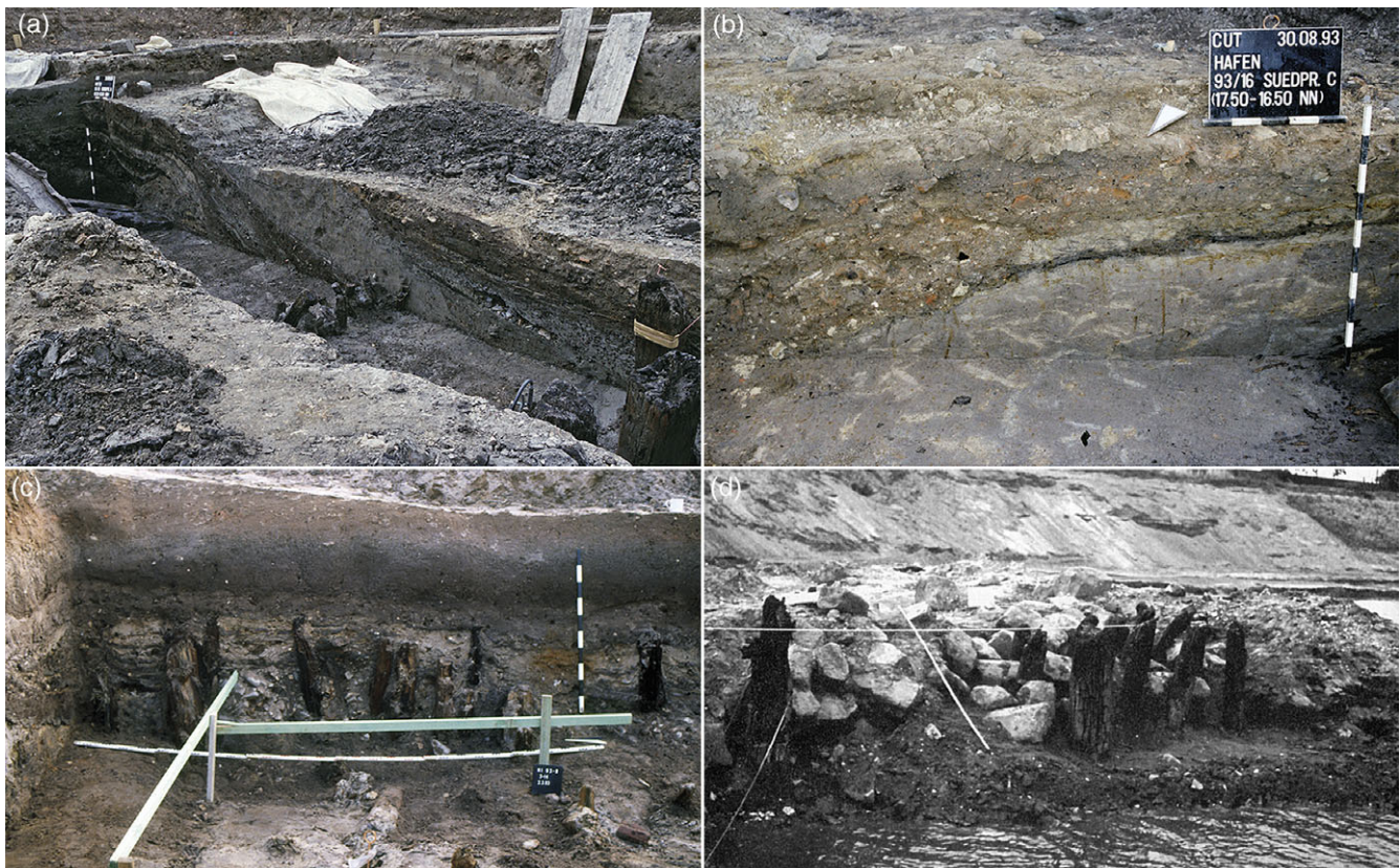
Fig. 13. Roman bank protection constructions. (a) Xanten CUT bank protection (“Packwerk”): square timber posts (right) and smaller piles in organic layers (dark) and light colored “Senkerde” (Gerlach et al., 2016a, photo: LVR-APX by Bernd Münster). (b) Xanten CUT bank protection: detail from the earthen construction (below): the individual loamy spade clods ( caespites ) can still be recognised by the light stripes that correspond to the former humus top soil (Gerlach et al., 2016a, photo: LVR-APX by Bernd Münster). (c) Moers-Asberg: rows of piles and soil infill (Gerlach et al., 2016a, photo: LVR-ABR by Clive Bridger, NI 1993/0008). (d) Krefeld-Gellep: rows of piles with basalt stone fillings (Meurers-Balke et al., 2015: 239, fig. 1, photo: Stadtarchäologie Krefeld).
