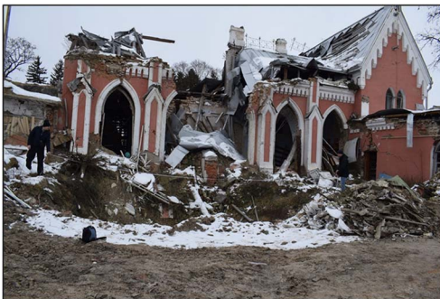
Figure 2. Children's Regional Library, former Vasyl Tarnovsky Museum of Ukrainian Antiquities, Chernihiv, Chernihiv Oblast, March 2022. Since bombing, the building has largely been unroofed, with the inside of the building left exposed to rain and snow (figure by Viacheslav Skorokhod).
