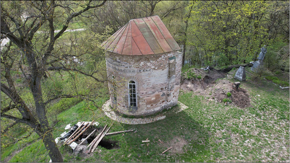
Figure 5. Standing remains of eleventh-century Каплиця Святого Юра (St George Chapel), Oster, Chernihiv Oblast, Ukraine, April 2023. To the left of the chapel is a partially covered bunker and on the right is a large trench that has dug through the brick foundation of the building (figure by Archaeological Landscapes Monitoring Group, 2023).
