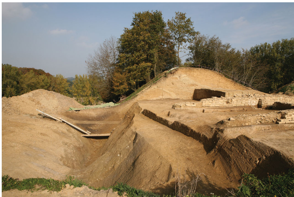
Figure 3. Monumental stone gate forming the entrance to the lower town of the Heuneburg: profile through the bank, stone gate pedestal and ditch (©Landesamt für Denkmalpflege).
