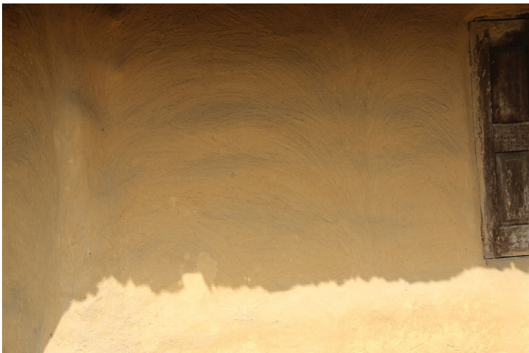
Figure 6. Idu-Èkpèyè village. Stucco wall after plastering with clay. Photo by the author, 2017.
