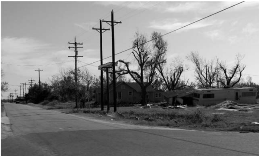
Figure 2.23 High Island, Texas, after Hurricane Ike.
