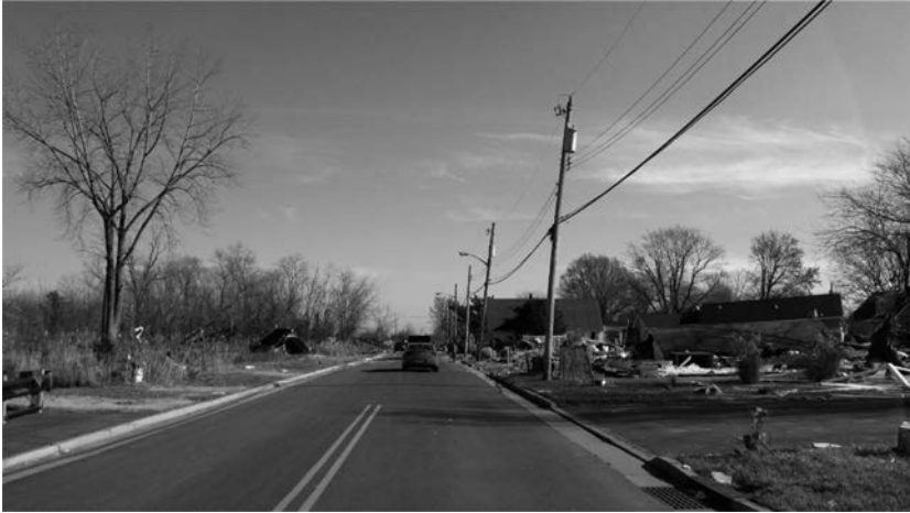
Figure 2.24 Union Beach, New Jersey, after Superstorm Sandy.
