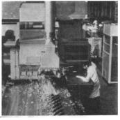
BAC's method of machining skin panels from solid metal slabs involves up to 80 per cent of the metal being cut away
