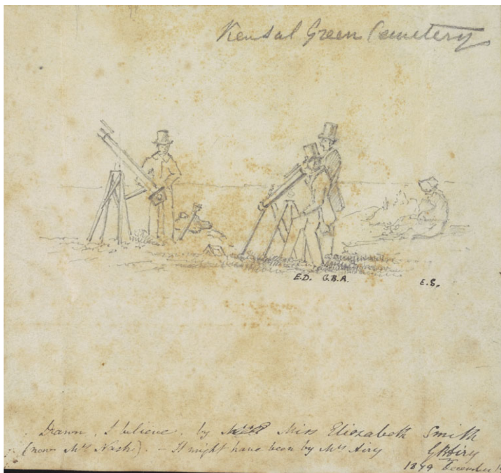
Figure 4. Drawing of collimator experiments in Kensal Green Cemetery, with Airy to the right of the observer employing the telescope. Airy noted on 19 December 1879 that this was drawn either by his wife Richarda Airy or by her sister Elizabeth Smith (later Elizabeth Nash). Loose drawing in RGO/6/47. Reproduced by kind permission of the Syndics of Cambridge University Library.
