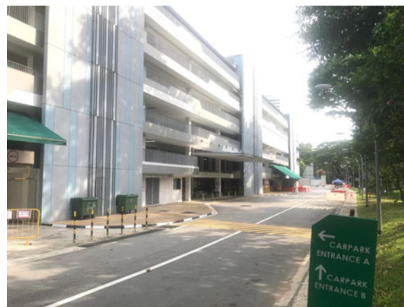
Multi-story Carpark (MCSF).
