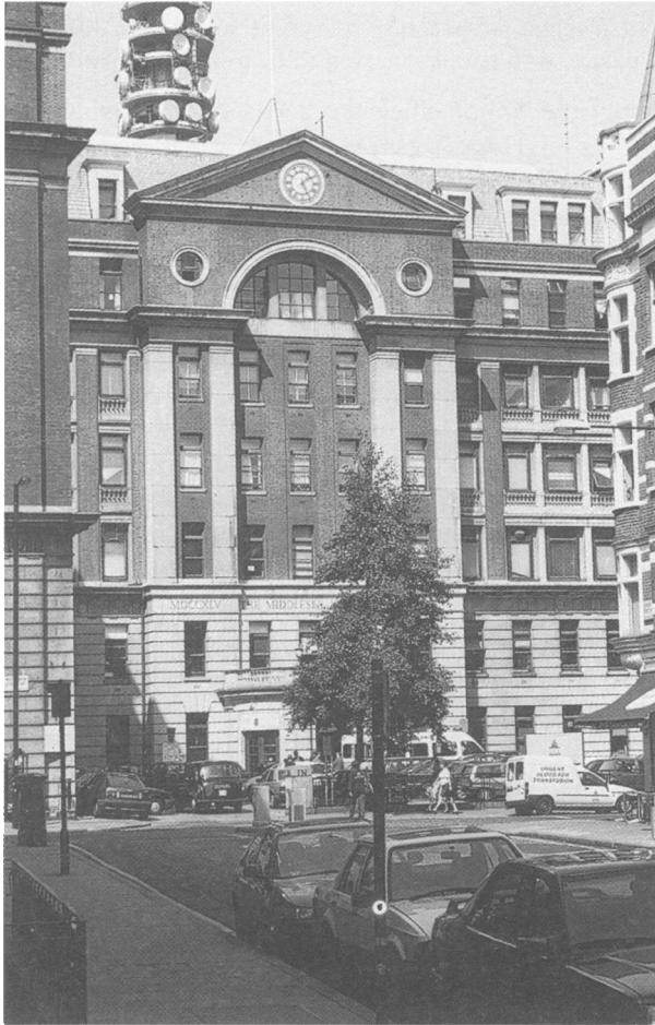
Figure 8: Middlesex Hospital, Fitzrovia, London, Alner Hall, 1926–35. (Photo: Jonathan Hughes.)
