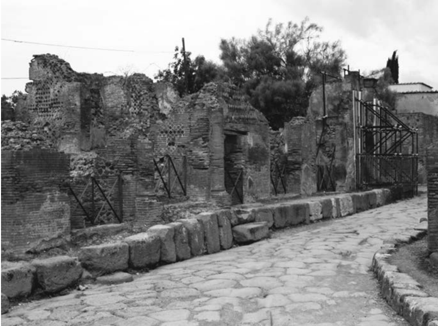
28. Across the frontage of the Casa di Diana II in Pompeii (VI.17.32–38) ran an elevated sidewalk that lifted the house and caused an inconvenience for pedestrians.
