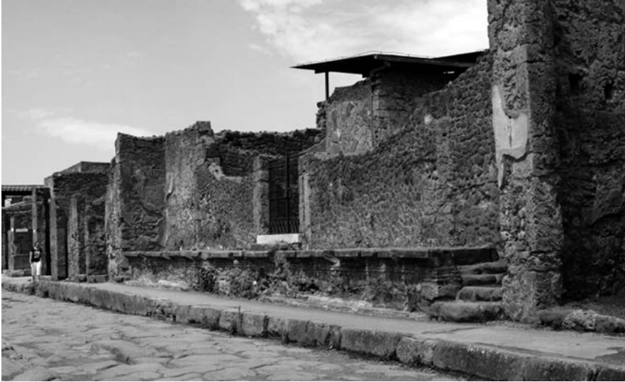
31. The Casa di M. Epidius Rufus at Pompeii (IX.1.20) was lifted above neighboring structures atop a temple-like podium, which supported a secondary sidewalk.
