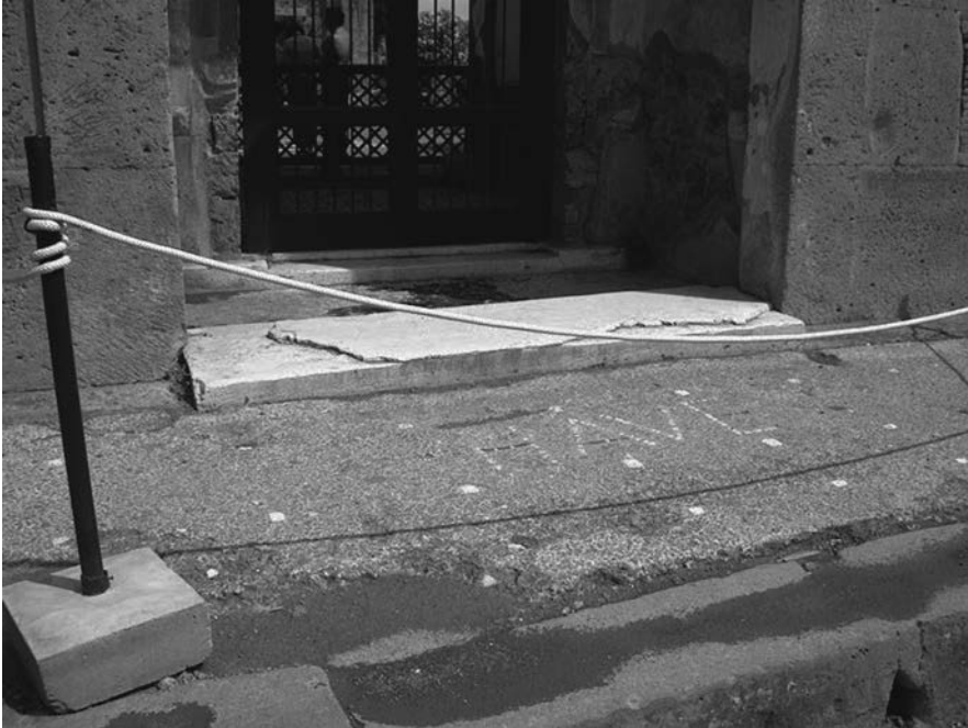
27. The sidewalk in front of the Casa del Fauno in Pompeii (VI.12.1–6) consisted of a grid of white marble chips set in a black matrix, along with a polychrome greeting, “HAVE,” spelled in front of the house’s main entry.
