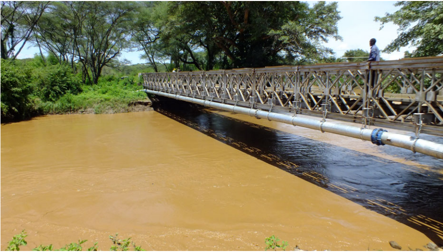
Figure 4. The Tot-Kolowa main pipeline crosses the Kerio River, attached to the main road bridge.
