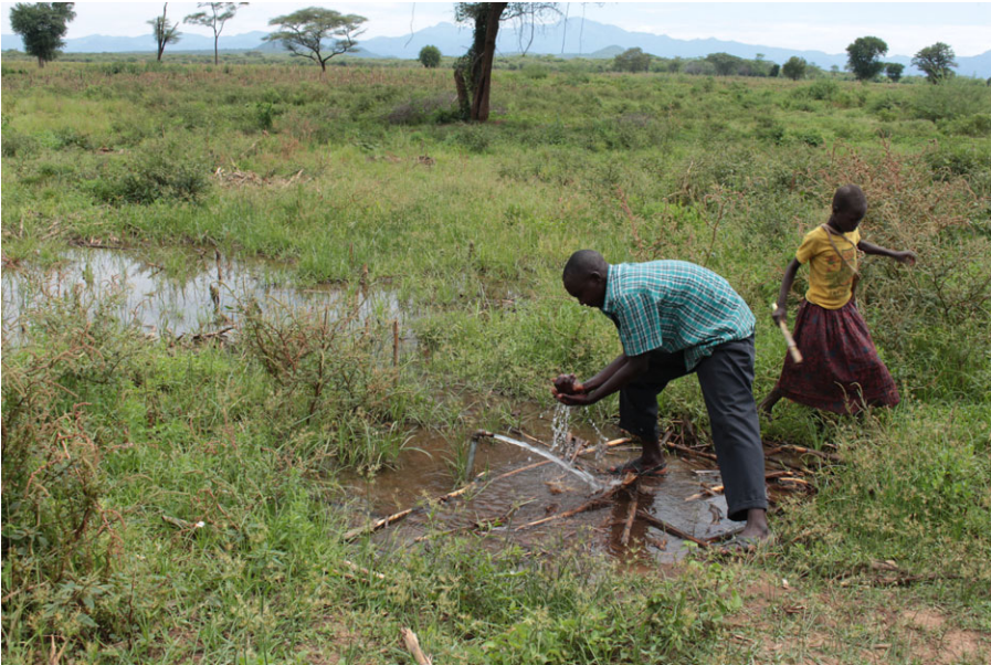
Figure 8a. Water pooling on the Pokot side due to a missing tap and improper control of cut-off valves.
