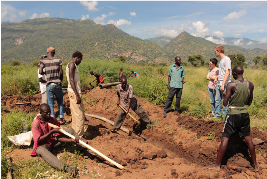
Figure 6. Work team repairing a pipe junction in 2014.
