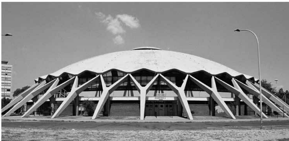
11 Top: The Palazzetto dello Sport of Rome designed by Pier Luigi Nervi (1957–60). Bottom: section of the Nervi's dome with detail of the spring featuring a full architectural integration with its supporting strut.
