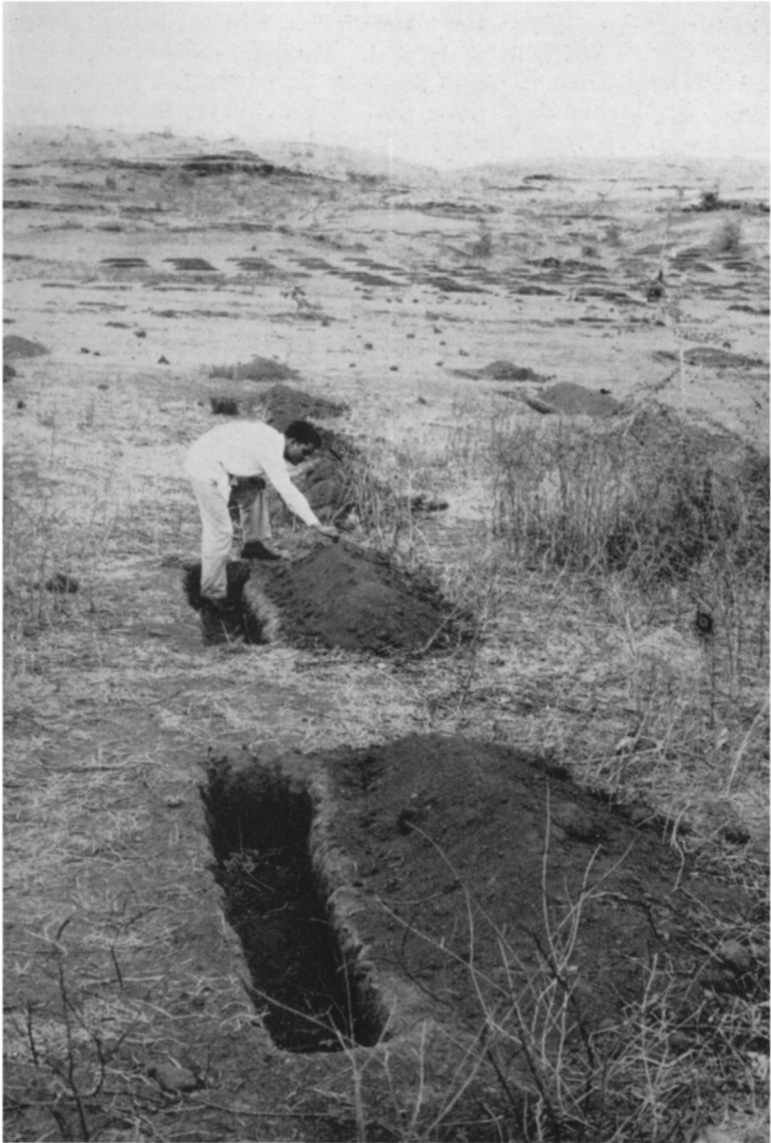
FIG. 13. —Ditch-and-berm planting and erosion control technique. Ditches are dug across the slope with the earth piled at the lower edge to form the berm. Tree shoots are planted in the loose earth.
