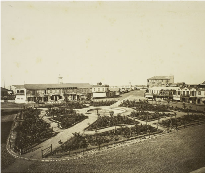
Figure 1. “View of La Place de Lesseps in Port Said,” photograph by Hippolyte Arnoux (1869, prior to the inauguration of the canal). Visible at the center is the planned square, park, and fountain demonstrating the Suez Canal Company’s ability to pipe fresh Nile water to canal cities. Harvard Fine Arts Library, Special Collections Valer and Olga Fricke album of photographs of the Middle East HSM:83:012:035 AKPI28.19.
