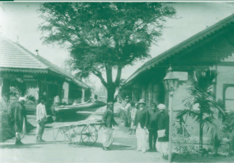
Plague Hospital, Bombay 1922. The disease was first acknowledged in Bombay in 1896, and only went into decline in the late 1920s. Photograph from Bain News Service (the first new photography service founded by George Grantham Bain in 1898). Glass negative preserved in Library of Congress, Washington D.C. Signature: LC-B2- 69-14 (P&P).
