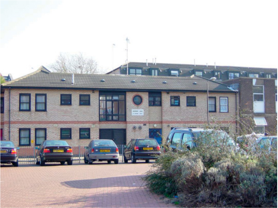
Figure 26.2 Thames Reach housing project, Bermondsey, 1994
